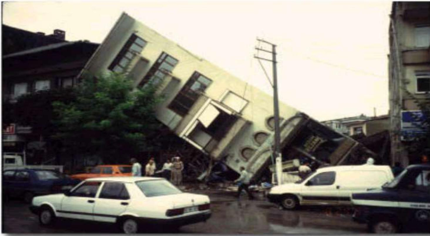
**The Izmit, Kocaeli, Turkey earthquake of 17 August, 1999, liquefied the soil beneath this apartment building's shallow mat foundation by reducing the bearing capacity to zero.**
