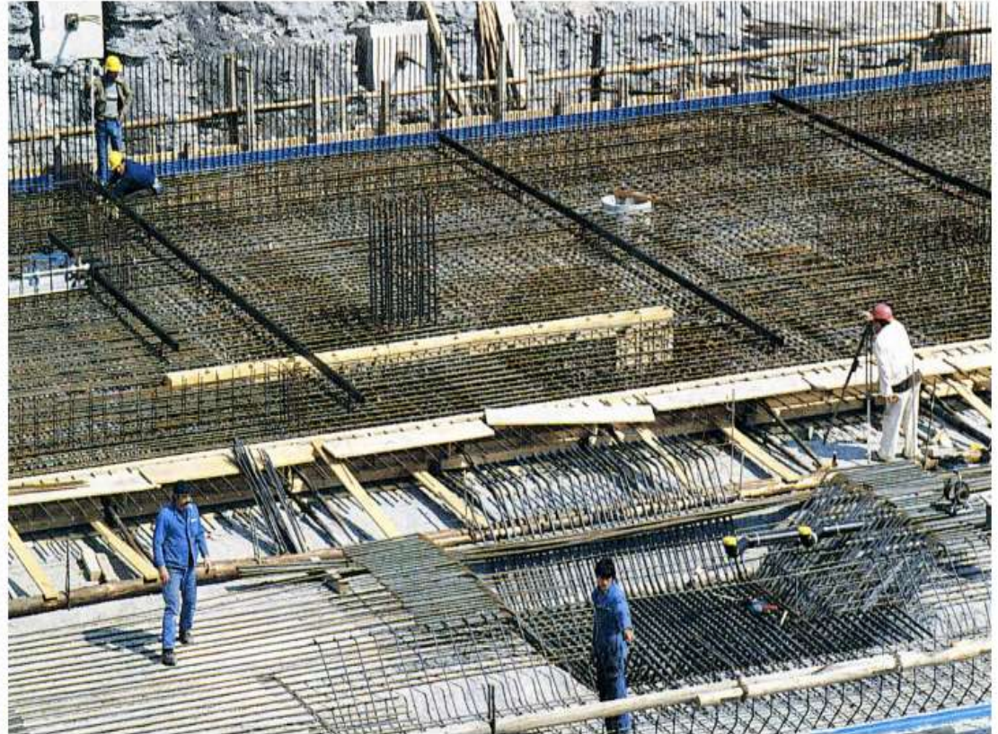
Large mat foundation in Switzerland.
