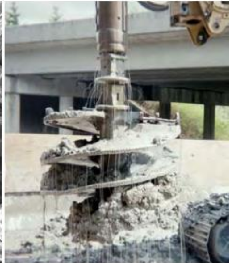
b) Polymer Slurry in Use
