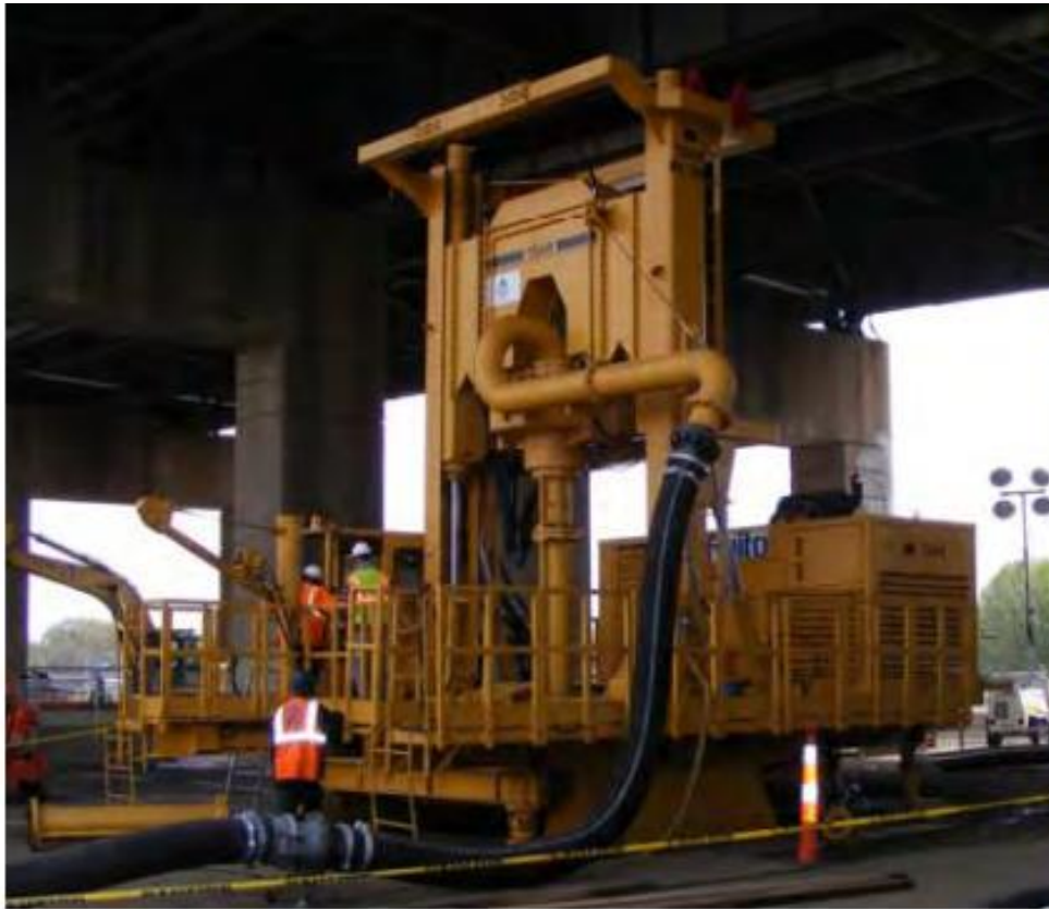
a) Restricted Headroom Drilling
