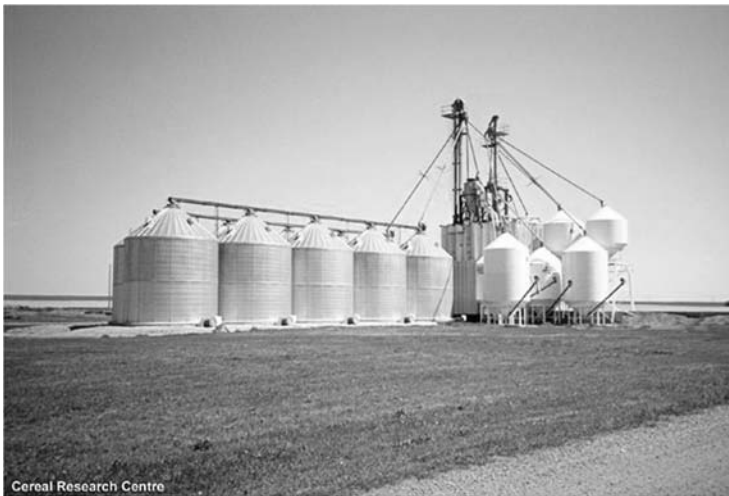
FIGURE 4.40 Storage bin complex. (From CRC. Agriculture and Agri-Food Canada. Winnipeg: Cereal Research Center.)
