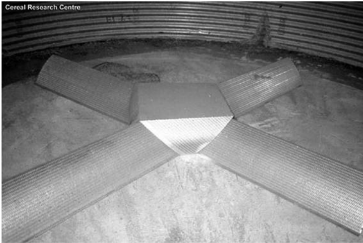
FIGURE 4.50 Aeration ducts in a bin. (From CRC. Agriculture and Agri-Food Canada. Winnipeg: Cereal Research Center.)
